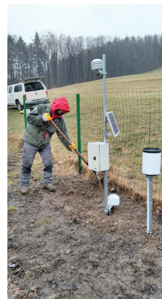
Installation of automatic climatic and environment monitoring station (CZ)
